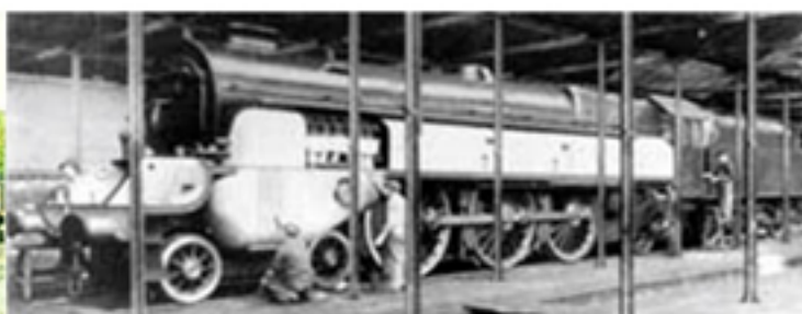
6202 having the cover for the forward turbine removed.
