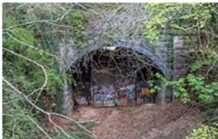
Walnut Tree (Garth) Tunnel South portal above.
